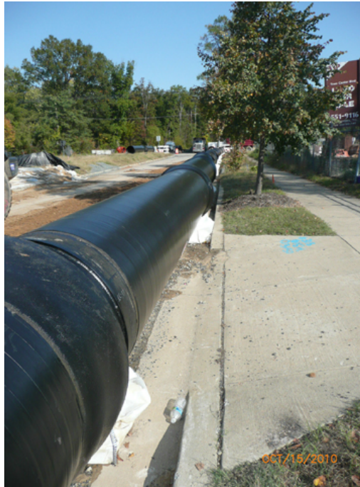
Figure 63 Tight-Bonded Ductile Iron Pipe Project October 2010 East Coast
