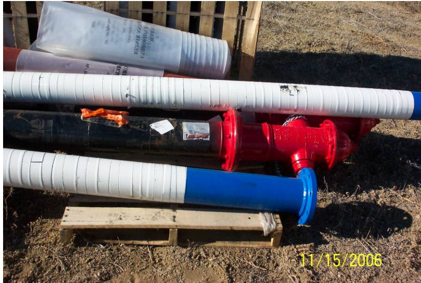
Figure 54 2006 Hand Taping of Ductile Iron Stub Pieces with FBE Fittings
