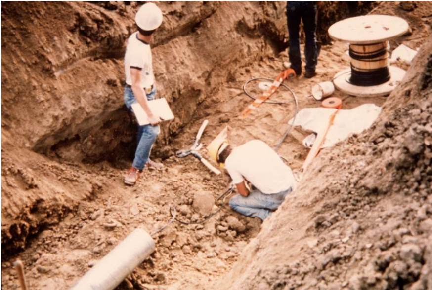
Figure 35 Denver, Colorado, Distributed Impressed Current Anode System for Dual Force Mains (103 to 137 Micro-Amps/Square Foot Current Requirement)
