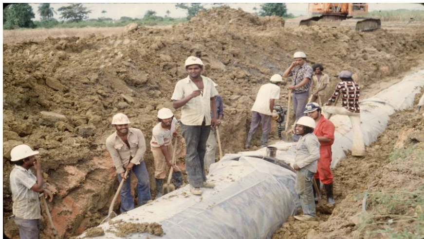
Figure 36 Trinidad-Tobago Polyethylene-encased Ductile Iron Pipe High Current Requirement in Low Resistivity Salt Contaminated Soils (>700 Micro-Amps/Square Foot)
