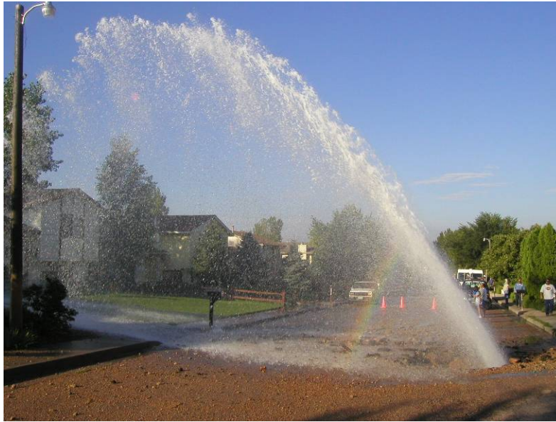
Figure 10 Major Leak on 24-Inch Polyethylene-encased Ductile Iron Line in Colorado
