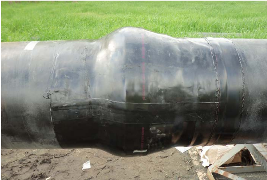
Figure 66 High Recovery Heat Shrink Bore Kit Sleeve
