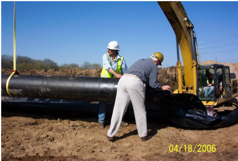
Figure 44 Inner Layer of 8-mil Anti-MIC Polyethylene Encasement
