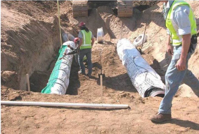
Figure 47 Polyethylene-encased Ductile Iron Ribbon Anode Cathodic Protection System
