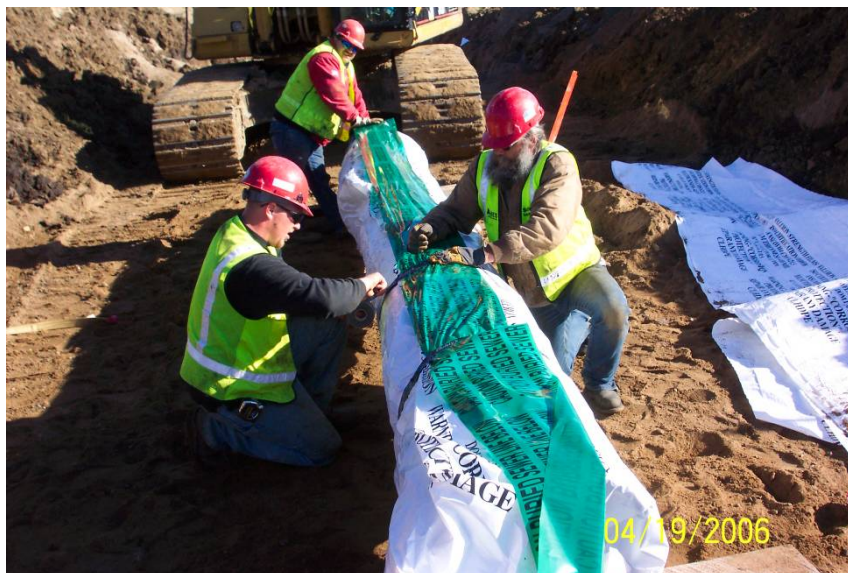
Figure 45 Folding Over of 4-mil Outer Wrap of High-Density Cross-Laminated Polyethylene Encasement and Taping In Place With Identification Tape
