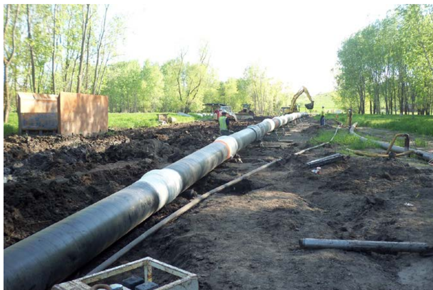
Figure 68 Tight-Bonded Coated Ductile Iron Bore Pipe Ready to be Pulled Under River
