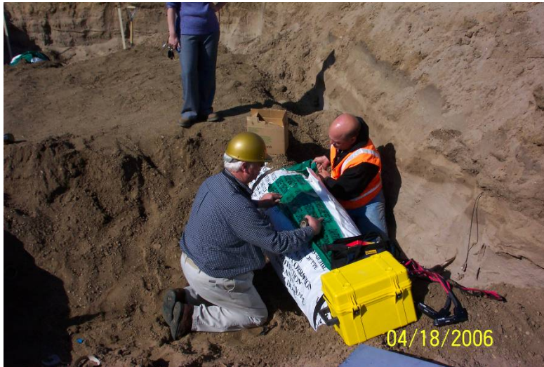
Figure 46 Joint Bonded and Polyethylene Encasement Overlap at Joint
