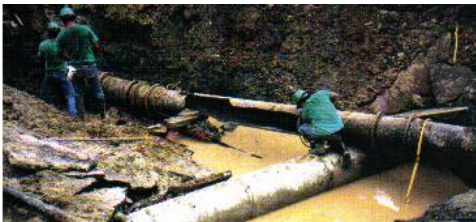
Figure 9 Catastrophic-Type Break Hawaii 34-Year-Old Cast Iron Main Break (14.5 Points)
