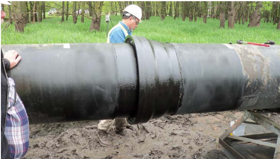
Figure 65 Heat Cured Epoxy Primed Ductile Iron Joint
