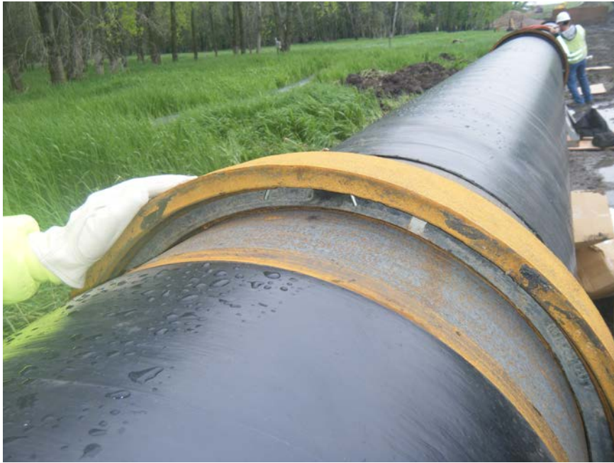
Figure 64 Tight-Bonded Coated Internally Restrained Ductile Iron Bore Pipe 2011
