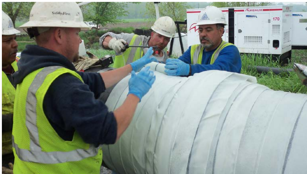
Figure 67 Water Activated Glass Impregnated Protective Sleeve at 50% Overlap 6 to 8 Layers
