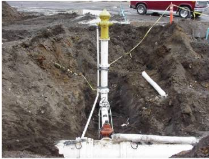
Figure 60 Seattle Thermoplastic Coated Cathodic Protected Ductile Iron Pipe With Fusion-Bonded Coated Fittings
